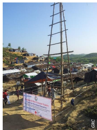
Drilling of borehole in the camp.
