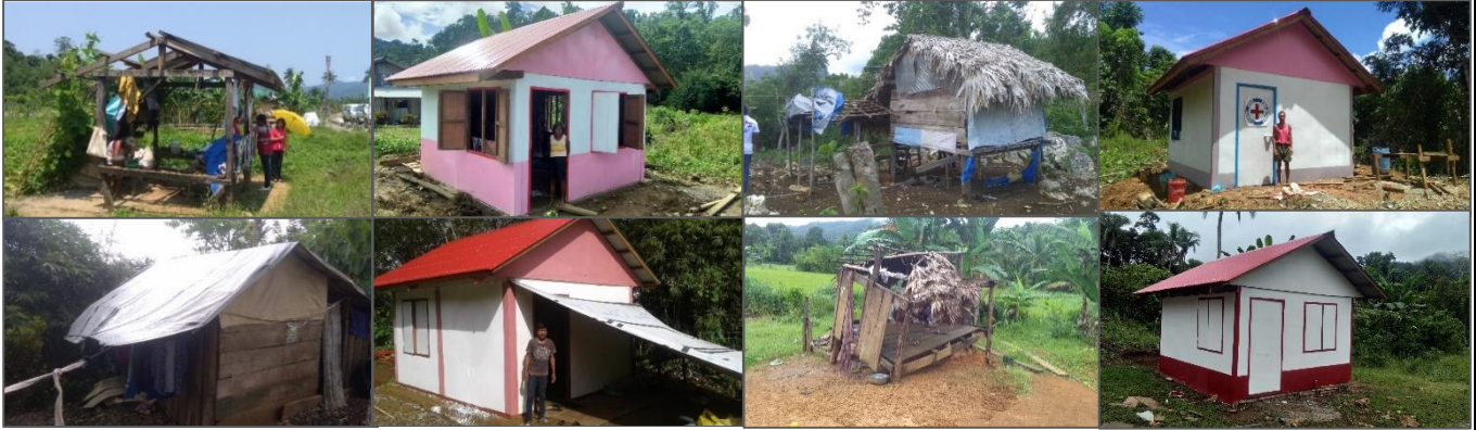
Some before and after photos of the shelter. (Photo: PRC/IFRC)
