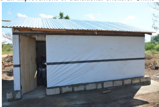
Completed Temporary Shelter
