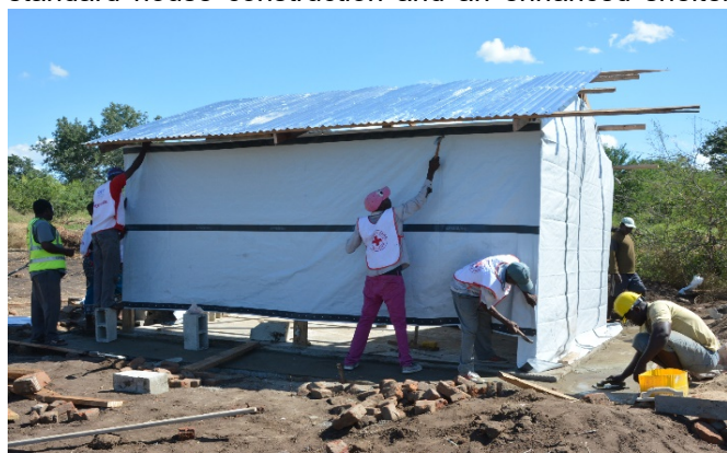
Construction of Shelter in Chikwawa District
