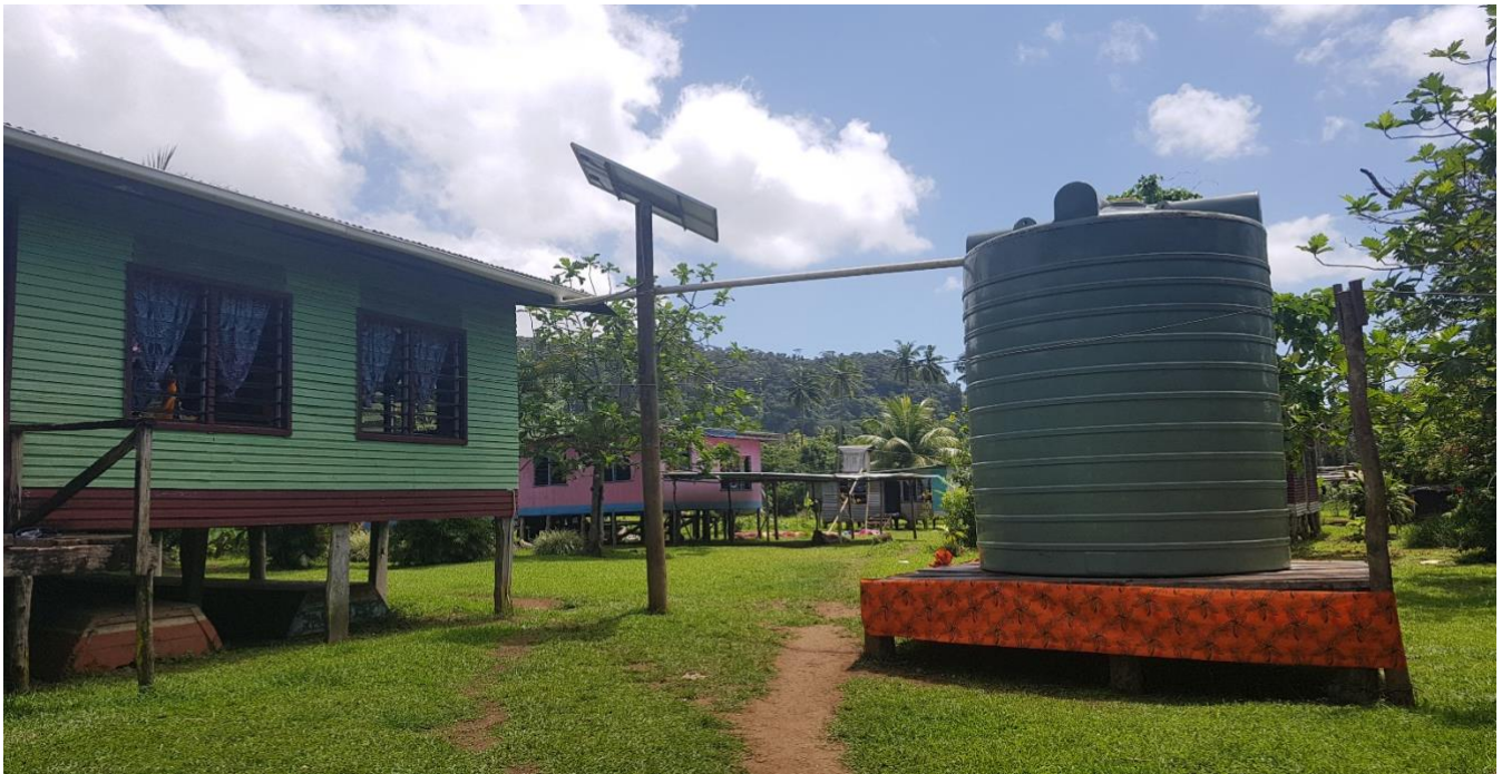
Rainwater harvesting connection to the BRCF supported water tank at Naiqaqi Village, Savusavu. Photo Credit: Iris Low
