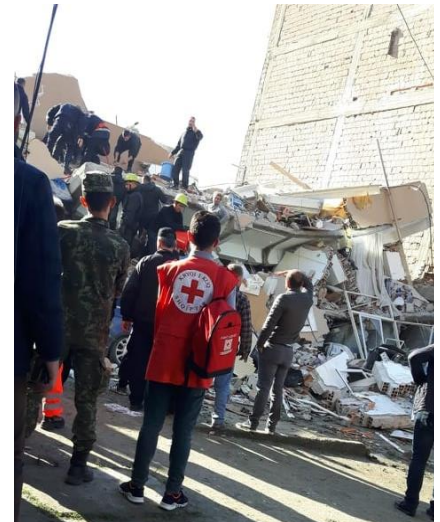
A volunteer at the ruins of a building collapsed during the earthquake in Durres. Photo: Albanian Red Cross
