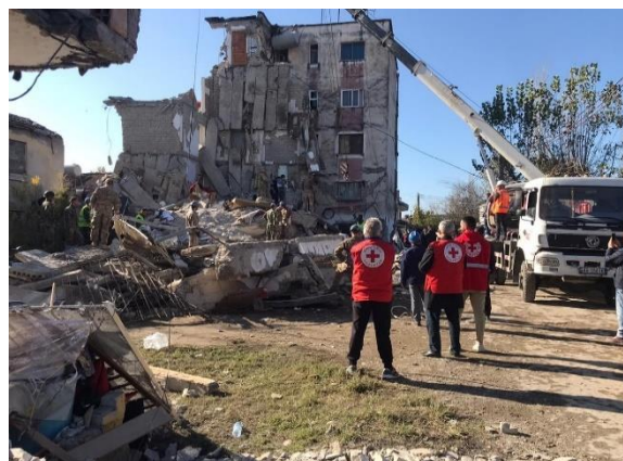
Image 1 - Collapsed building in Durrës. Photo:
