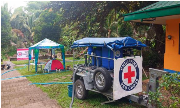
Set up of water filtration unit. (Photo: PRC)
