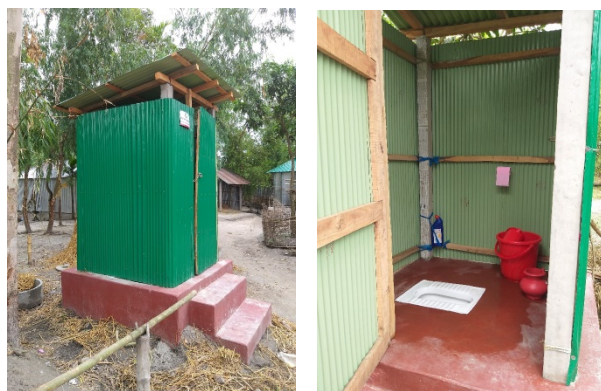
Figure 9: (left) A latrine with a raised toilet base. Right (interior condition of the latrine – which looks clean and has a few hygiene materials) (Photo: IFRC)
