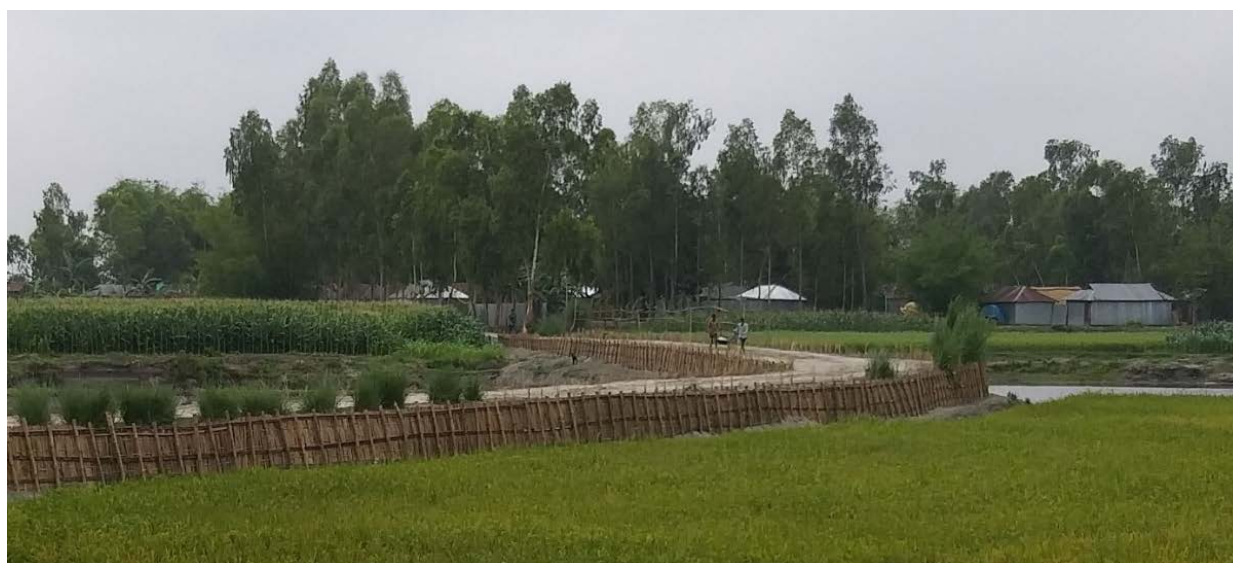
Figure 10: A constructed road with palisade placed on both side of the road, to minimize flood impact (Photo: IFRC)
