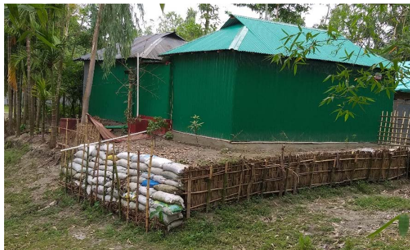
Figure 8: Newly constructed shelters. (Photo: IFRC)
