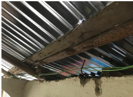
Photo: Laminas installed on wood in bad condition
