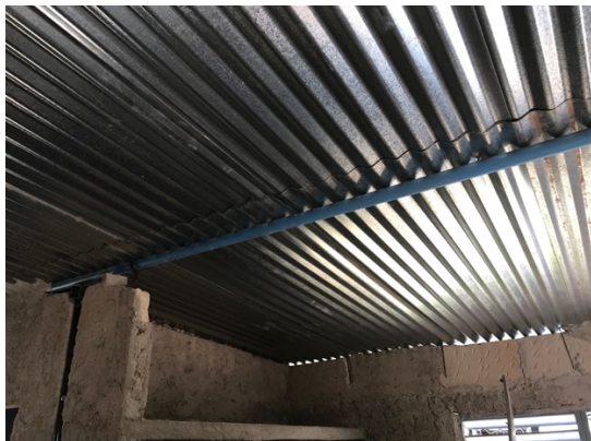
Photo: Sheets installed on plastic bars
