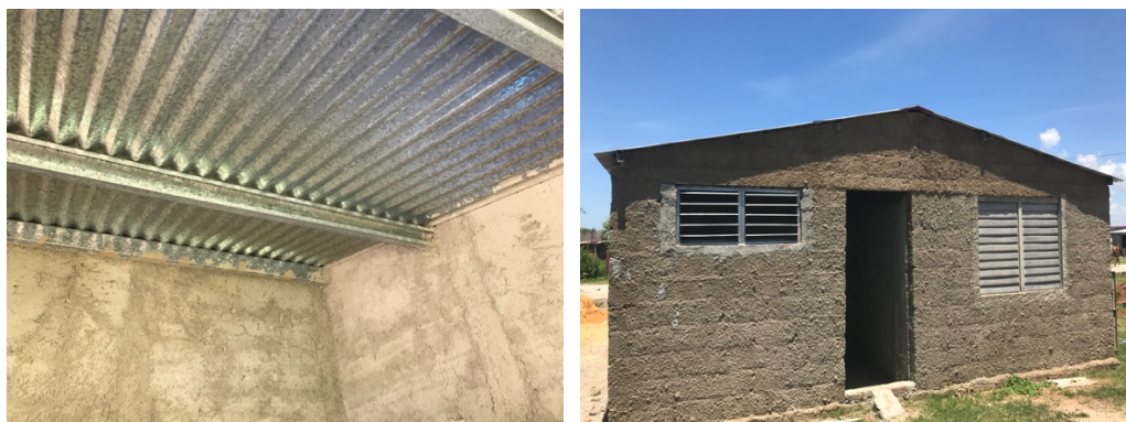
Photos: House with a roof installed on a metallic structure
