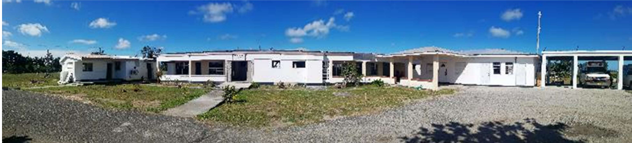
Hannah Hospital in Barbuda, with the main ward (central structure on picture) still being rebuilt.
