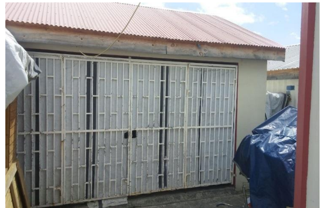
Figure 19- Warehouse outside DRCS Main Building
