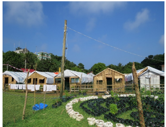
Temporary Learning Spaces Centre in Plaza ground. (Photo: Rajeev K.C. IFRC)
