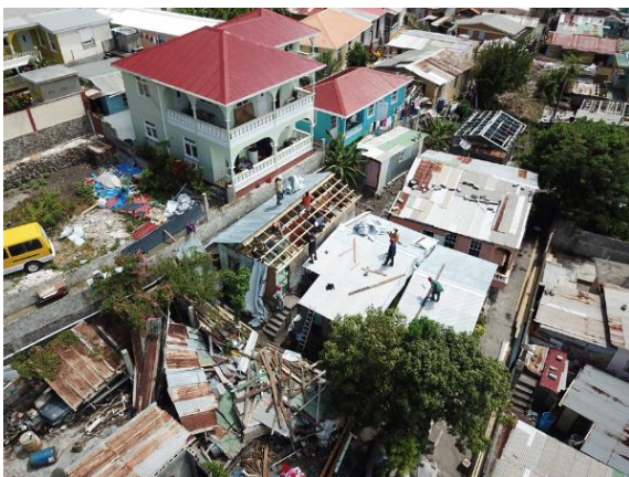
Photos: Left and right: Damaged roofs undergoing repair work in Dominica. Source: Dominica Red Cross Society (DRCS), 2018.
