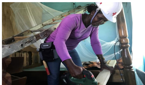
A DRCS volunteer repairs a damaged roof. Source: DRCS
