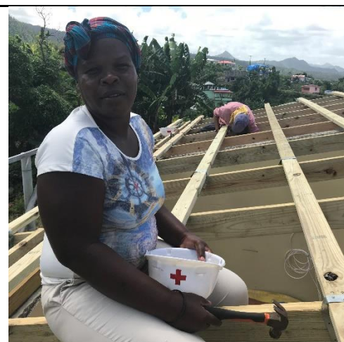
A DRCS volunteer repairs a damaged roof. Source: IFRC
