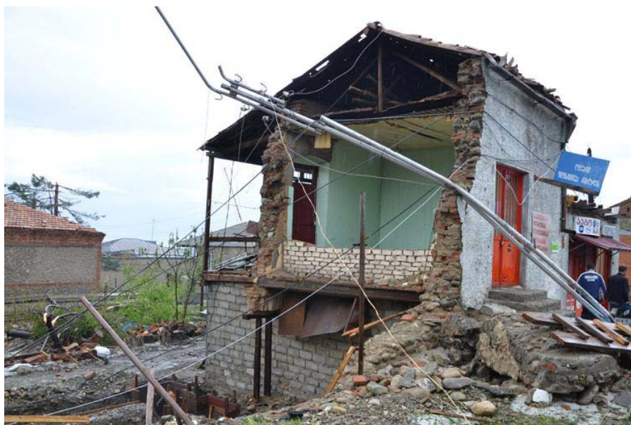
A residential building destroyed by the floods. Photo: Georgia RC
