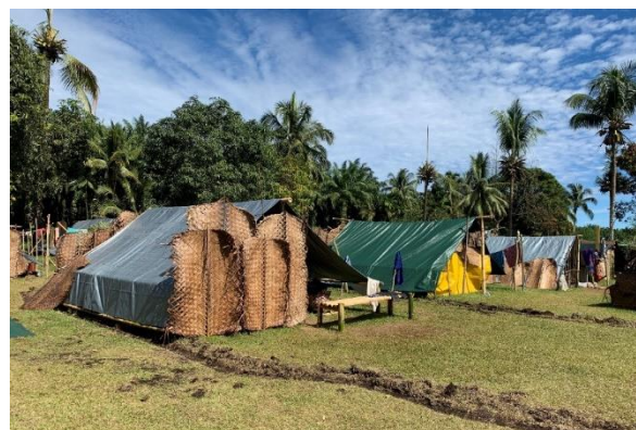
IDPs site with emergency shelters made of donated tarpaulins and locally available materials. (Photo: IFRC)
