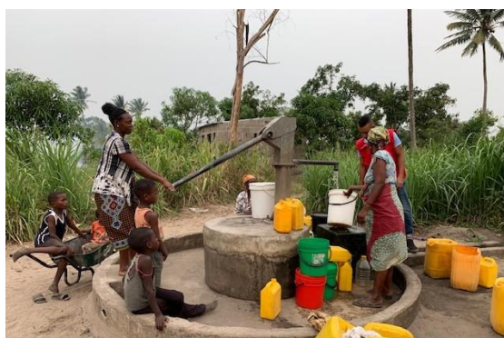
Image 4- Rehabilitated water pump in Ngupa, Beira district. Photo: IFRC
