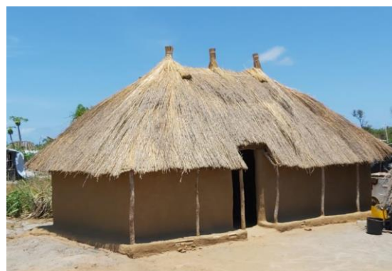
Image 1- Traditional house model built using local strengthened techniques. Photo: IFRC
