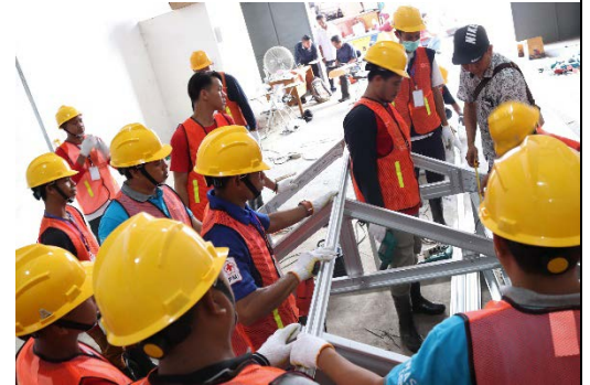
Masons and carpenters practicing joint technique for light steel during safe shelter training. (Photo: PMI)
