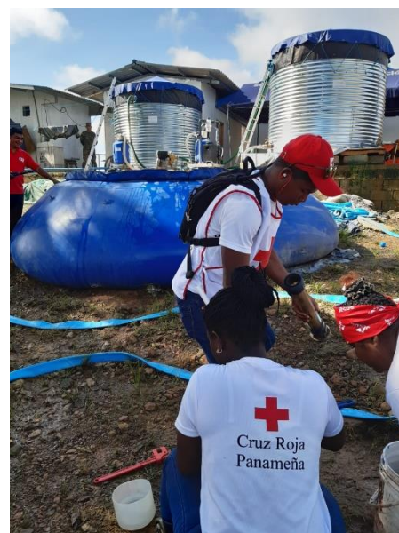
PRCS volunteers work on the water purification facility in Darien in November 2019. Source: PRCS
