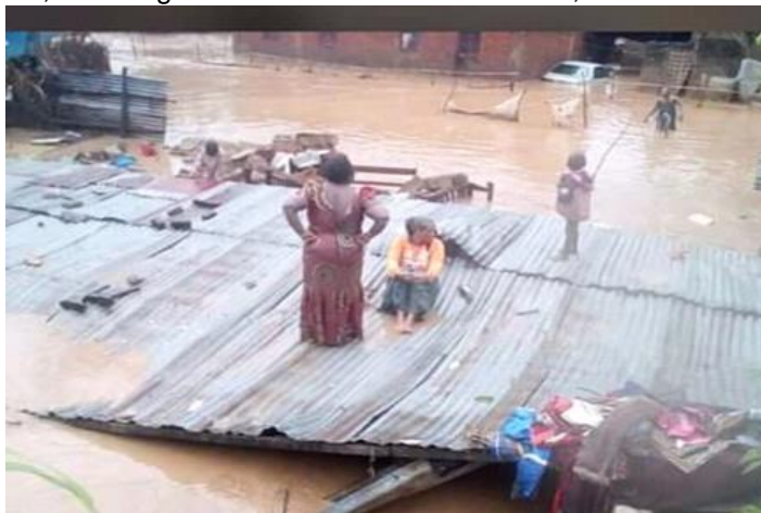
Affected family on the roof of their damaged and flooded house © DRC RC
