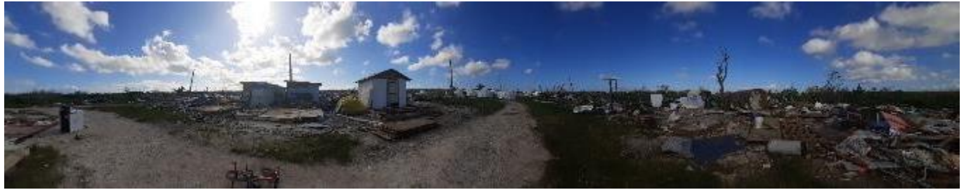
Photo 9: IFRC WASH Hydrogeologist jointly with the relief team conducted field visits to The Farm settlement in near Treasure Cay (Abaco) between October and November 2019. All houses in The Farm suffered severe damages with many were totally destroyed. Source: IFRC
