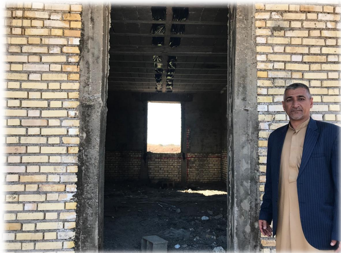
Figure 10. Cash used for reconstruction in Golestan– photo credit: IFRC
