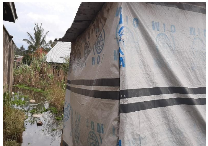
Picture 2: Flooded Makeshift structure erected during 2016 earthquake in Kagera.
