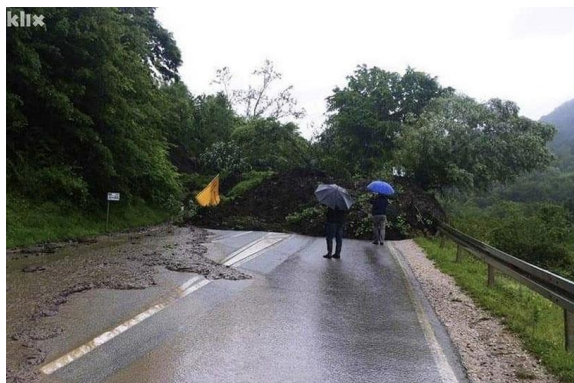
Image 1 - Landslide in Kladanj, Tuzla Canton. Photo: Klix.ba
