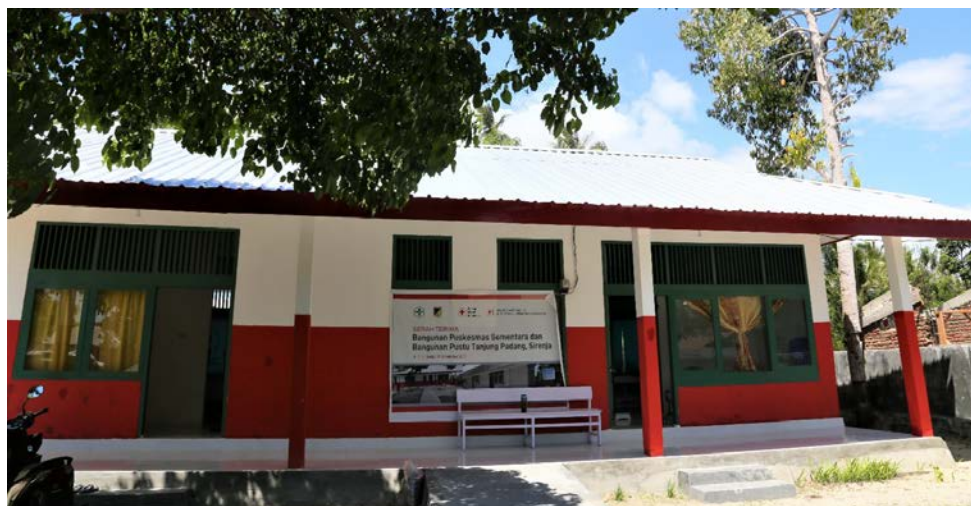
Rehabilitated Pustu in Tanjung Padang, Sirenja, Donggala. (Photo: IFRC)
