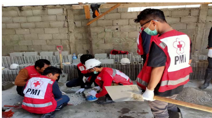
PMI volunteers trained on making blocks, which will be replicated with community members, to improve quality of shelter construction materials. (Photo: PMI)
