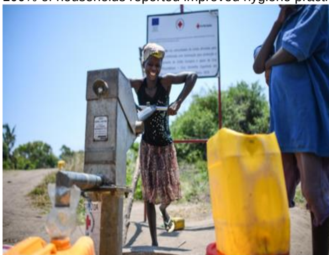
Rehabilitated Water Pump in Ngupa-Dondo
