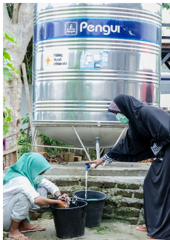
Access to water across the four operational districts have been enhanced through the support of PMI and IFRC. More than 150 water access points have been repaired and installed with 2,000 litre water tanks. (Photo: PMI/IFRC)
