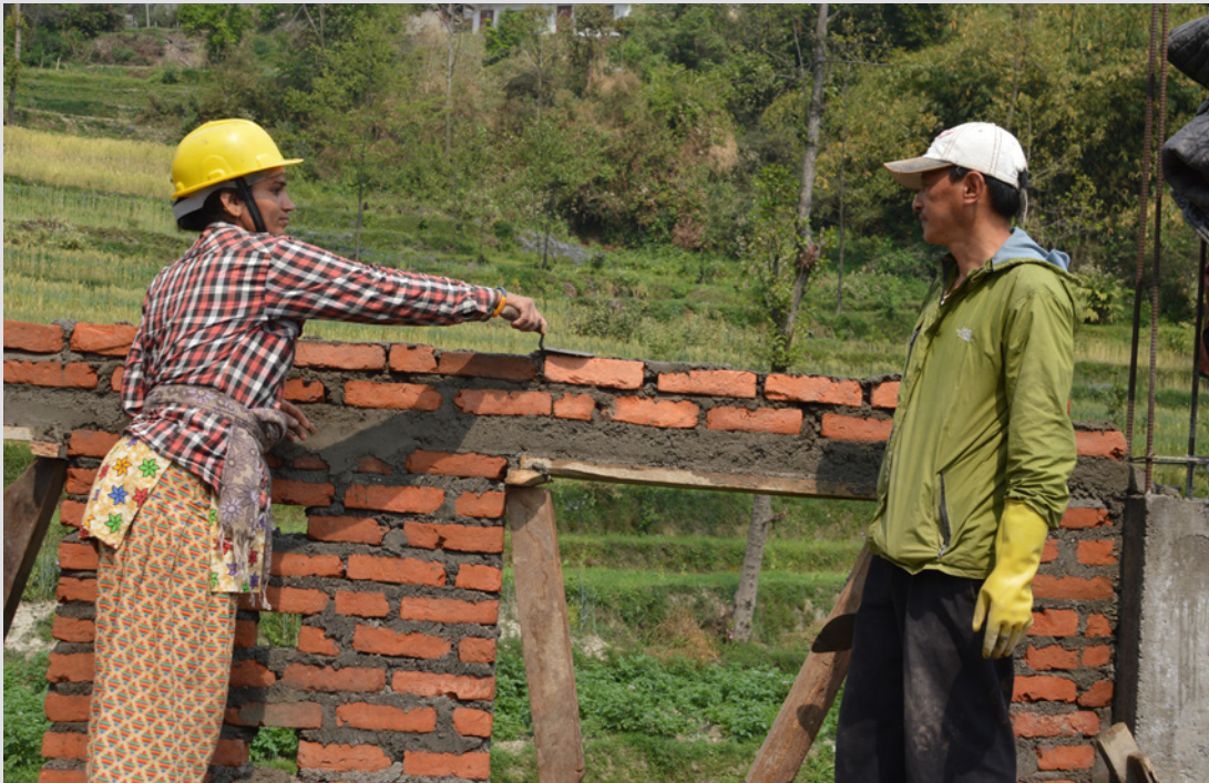
Huma placing bricks at a construction site. NRCS
