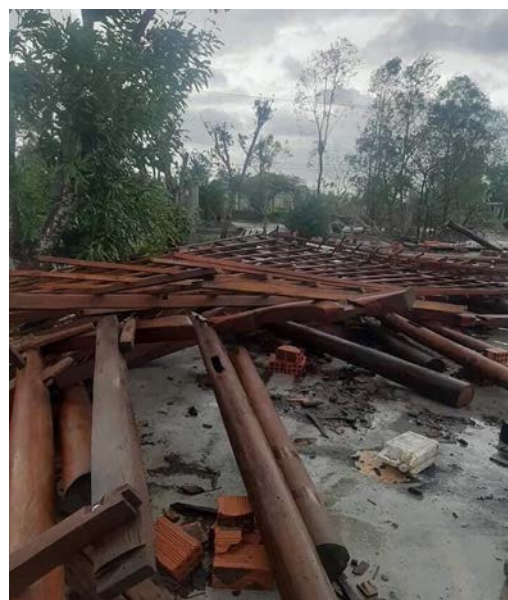
House totally collapsed in Quang Long district, Quang Binh province, 15 November. (Photo: VNRC Quang Binh Chapter)
