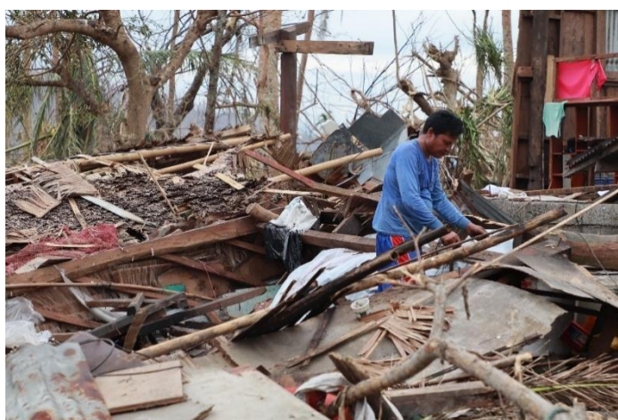
Houses damaged by Super Typhoon Goni (Photo: PRC)
