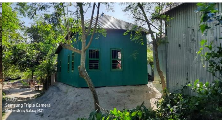
Beneficiaries has been constructing their houses by raising plinth in Sirajganj (left) and Tangail (right). (Photo: IFRC)
