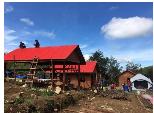
Houses are being constructed (Photo: IFRC)
