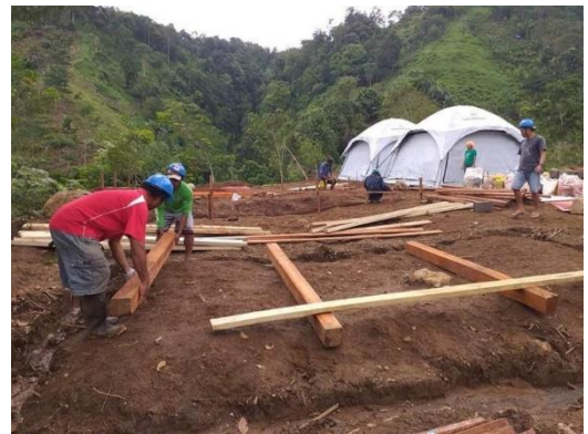
Ongoing construction in North Cotabato (Photo: IFRC)
