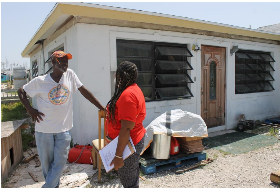
Photo 4: BRCS, IFRC and AmRC staff conducted a monitoring visit of the home repair programme in Abaco in November 2020 to assess progress and challenges. Source: Holly Baker, American Red Cross.
