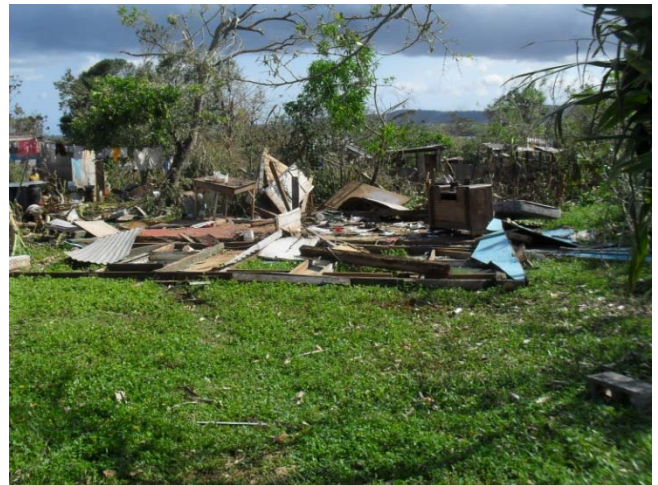
Hurricane Sandy led to destruction of homes and other infrastructure in Jamaica. Source: Jamaica Red Cross.
