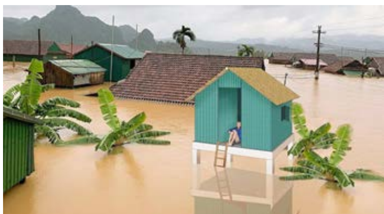
Illustration of a family evacuation shelter to be built beside existing houses if those housing are not strong enough to hold an attic or a mezzanine
