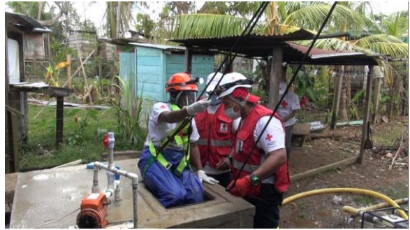
Well cleaning in affected communities on the Northern Caribbean Coast. Source: NRC, December 18, 2020
