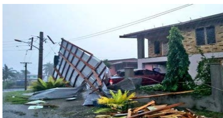
Photos of damage in Nasole, Nasinu (Central Division). (Photo: Fiji Village @ Legend)
