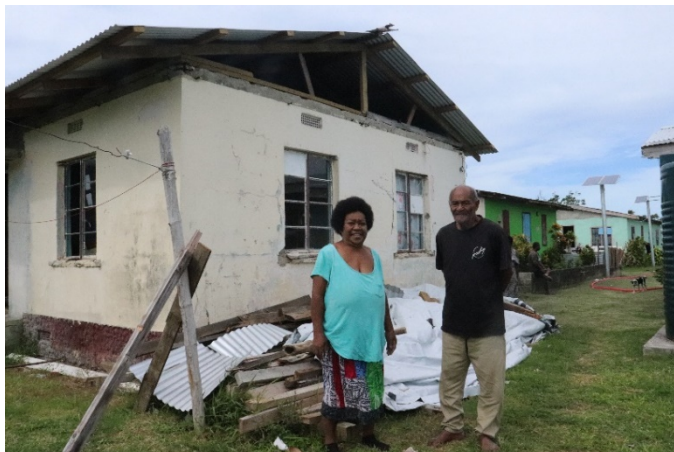
Iliesa standing with his wife beside their incomplete home. Building material of his house are seen behind him covered with the tarpaulin given by FRCS. (Photo: FRCS)
