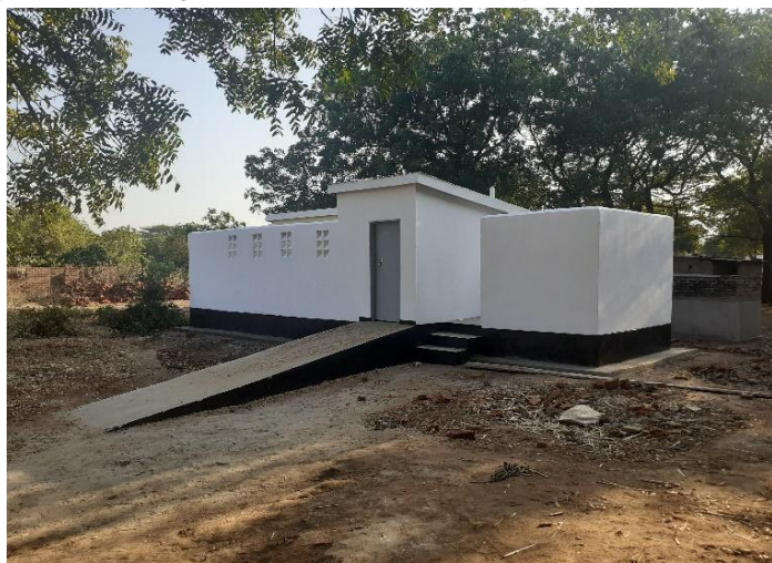
Rehabilitated latrine in Phalombe; Photo by MRCS
