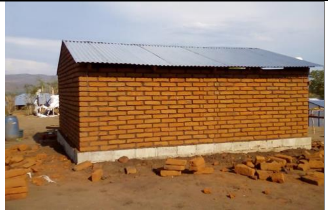
Figure 2 : Completed Permanent Shelter, photo credit: Malawi RC
