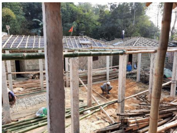
Mid-term shelters being constructed with durable concrete pillars in Camp 12 (Photo: IFRC)
