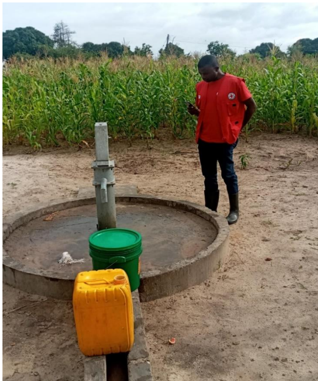
Water pumps recovery assessment by ZRCS staff
