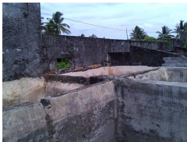
Large cistern layout ready for roofing cover PRG
