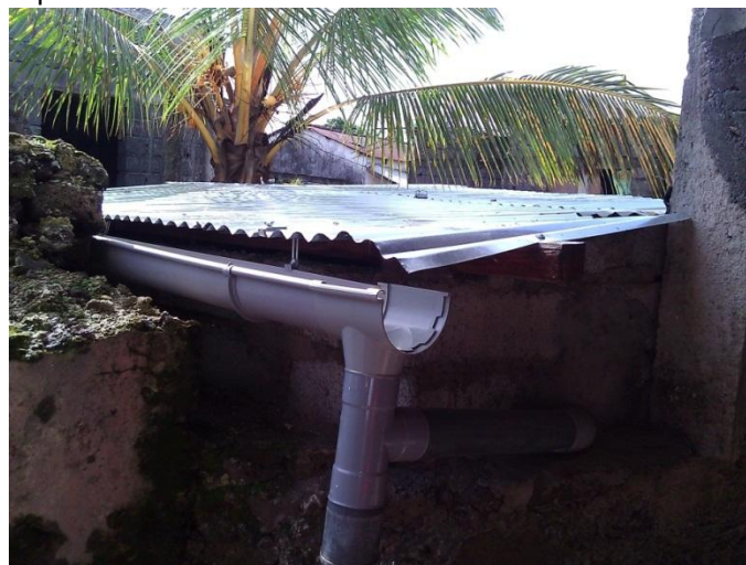
A repaired water cistern with guttering and roof PRG
