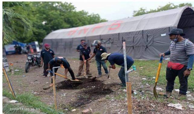
PMI volunteers digging infiltration holes at a temporary shelter in Kantor Bupati Lama. (Photo: PMI)
