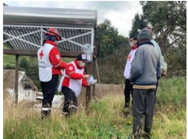
Photo 4. Installation of ashmetres, ERC
