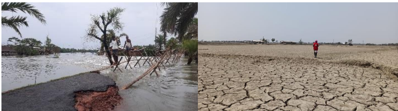
Due to cyclone Amphan impact, community infrastructure like embankment, road etc. damaged in coastal districts (Left photo: in Sathkira) and as consequence saline water intrusion, affected community lost their livelihood options like agricultural land. (Photo: BDRCS)
