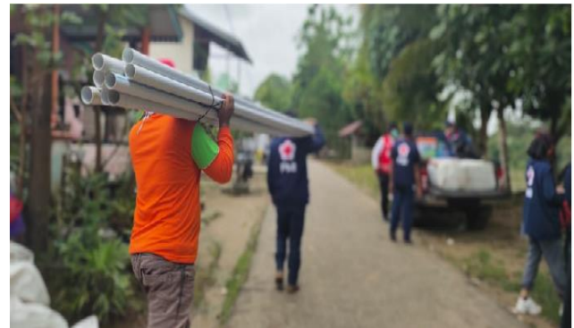
PMI rehabilitating damaged water line in Melawi. (Photo: PMI)
