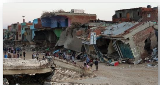
Figure 2 Damage of infrastructure from the floods. Credit: ERC
