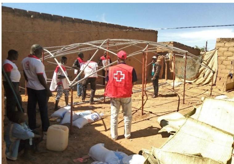
Burkina Red Cross volunteers supporting the construction of Sahel shelters @ BRCS
