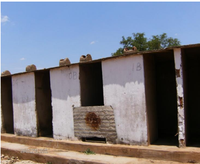
Picture 9: Old latrine block at Bethel Primary School.
