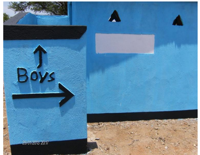
Picture 10: New latrines at Bethel Primary School.
