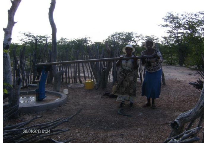
Picture 8: Rehabilitated water point in Matobo District.
