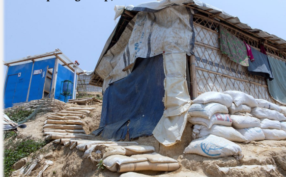
Sandbags shore up Mohammed and Roshida's shelter in Kutapalong camp, Cox's Bazar.
