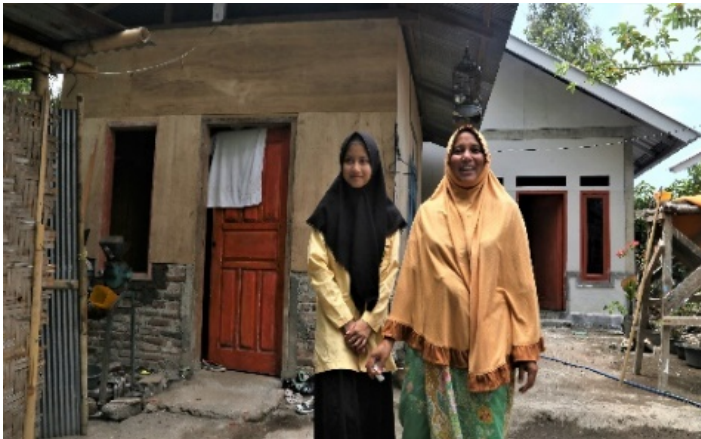
CVA phase 1 beneficiaries in North Lombok established semi-permanent houses utilizing plywood and iron roofing she redeemed with e-voucher provided by PMI. Photo: PMI/IFRC
