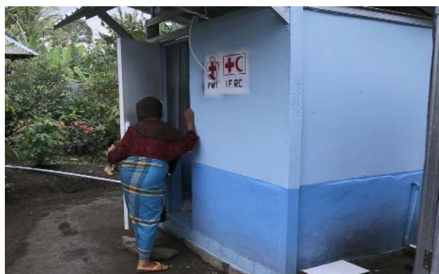
Prototype latrine constructed in a community as an example for proper latrine with septic tank construction. Photo: PMI
