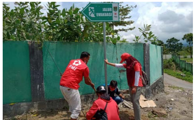
CBAT installing evacuation route mark in North Lombok. (Photo: PMI)
