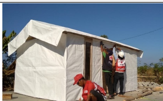
Emergency shelter construction for affected community in East Lombok. Photo: PMI
