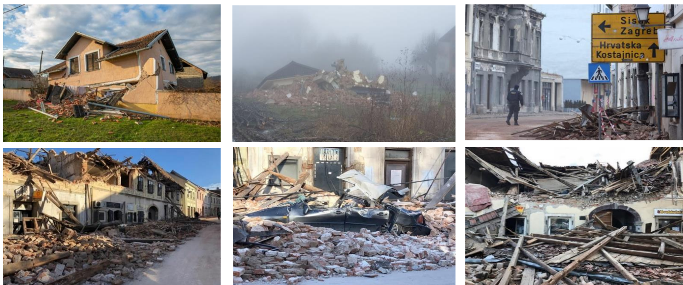
Image 1, 2, 3, 4, 5, 6: Photographs taken in the days and weeks following the earthquake on 29 December. There is still rubble and damage visible into late June, with reconstruction yet to take place.
