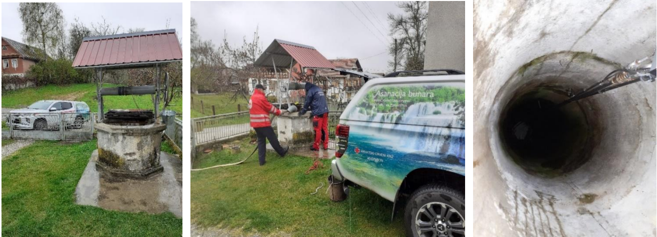
Image 31 & 32: Well cleaning in Sisak area. Source: CRC
